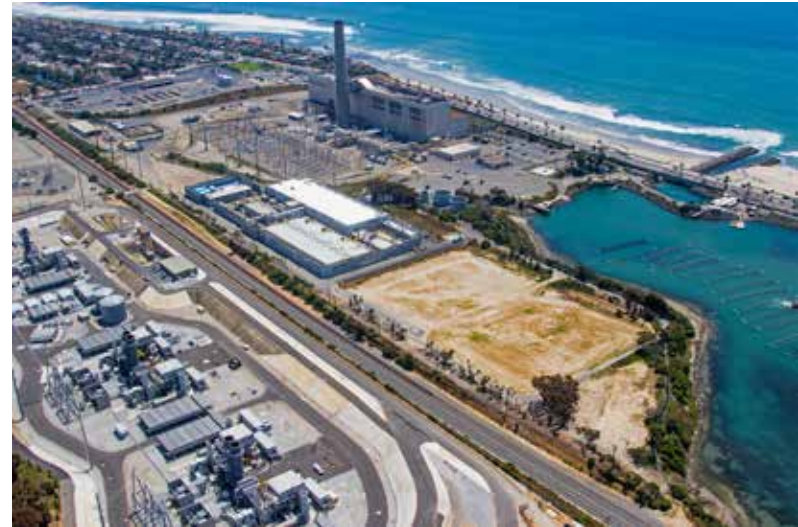
The Carlsbad Desalination Plant produces up to 54 million gallons per day of locally controlled water for San Diego County.
